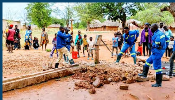
Community members take part in rehabilitating a dysfunctional hand pump in Luangwa District, Zambia to restore access to safe water.
